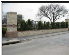
Combination of metal fence with masonry columns and base permits “openness” along the perimeter. Notice that extensive landscaping is included along the perimeter line.
