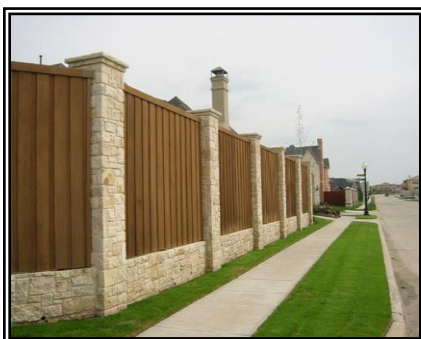
Combination of wood fences with masonry columns and bases is an appropriate fence. The capstones provide the vertical articulation. However, landscaping should be included as a part of any fence located along perimeter streets.
