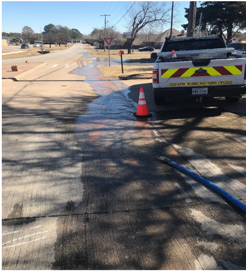
Atmos Crews – Water service hit during emergency gas repair (Backcharging for repair)
