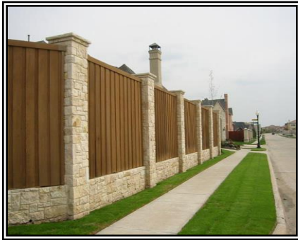
Example: Combination of wood fences with masonry columns and bases is an appropriate fence. The capstones provide the vertical articulation. However, landscaping should be included as a part of any fence located along perimeter streets.
