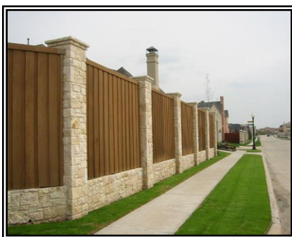
Combination of wood fences with masonry columns and bases is an appropriate fence. The capstones provide the vertical articulation. However, landscaping should be included as a part of any fence located along perimeter streets.
