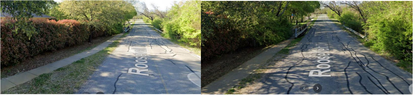
Heading north – shows change in sidewalk and existing guardrail
