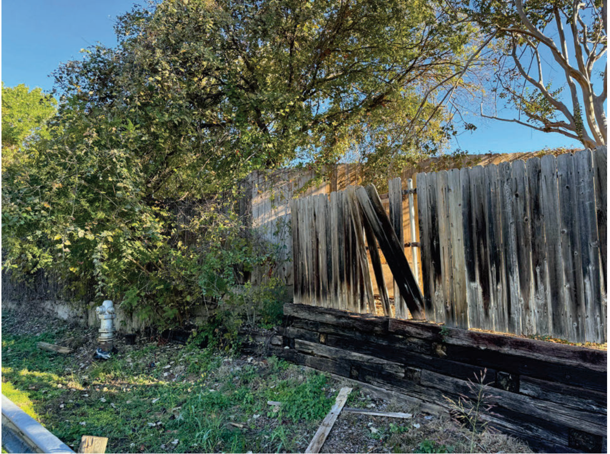
Another image of the fence at the corner of 3519 and 3520. The recent wind knocked down a few more boards.
