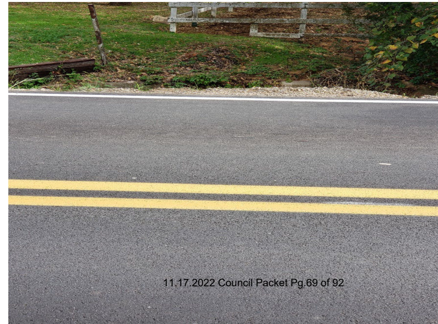
Looking East on Roosevelt (Box Culvert)
