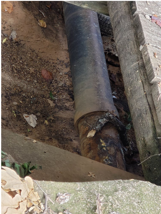
Slip Joint Coupling
