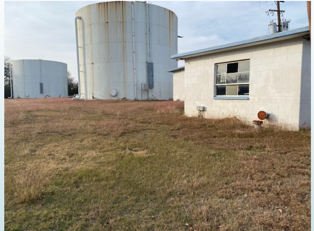
Both storage tanks to the west of pump station
