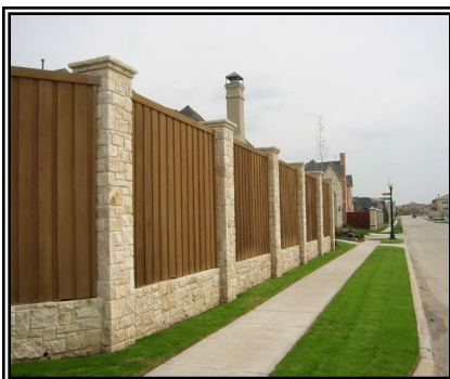
Combination of wood fences with masonry columns and bases is an appropriate fence. The capstones provide the vertical articulation. However, landscaping should be included as a part of any fence located along perimeter streets.
