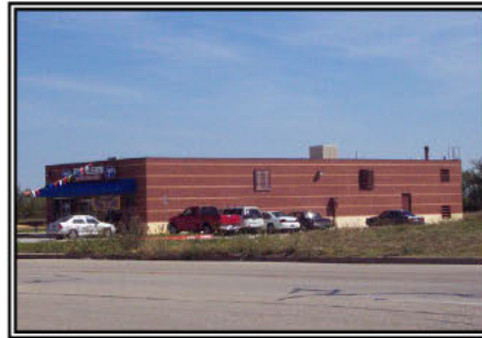
Lack of Articulation: Even extensive treatment of landscaping, awnings, and other frills cannot overcome a structure that has no variety in its horizontal and vertical surfaces
