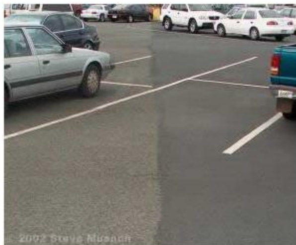
A parking lot shown with a fog seal (right) and without (left).
